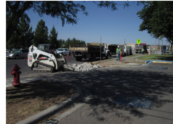
Work in progress at Valley View Elementary
